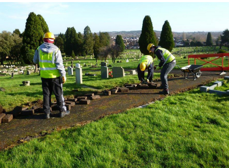
Skilled Up programme repairing pathways
