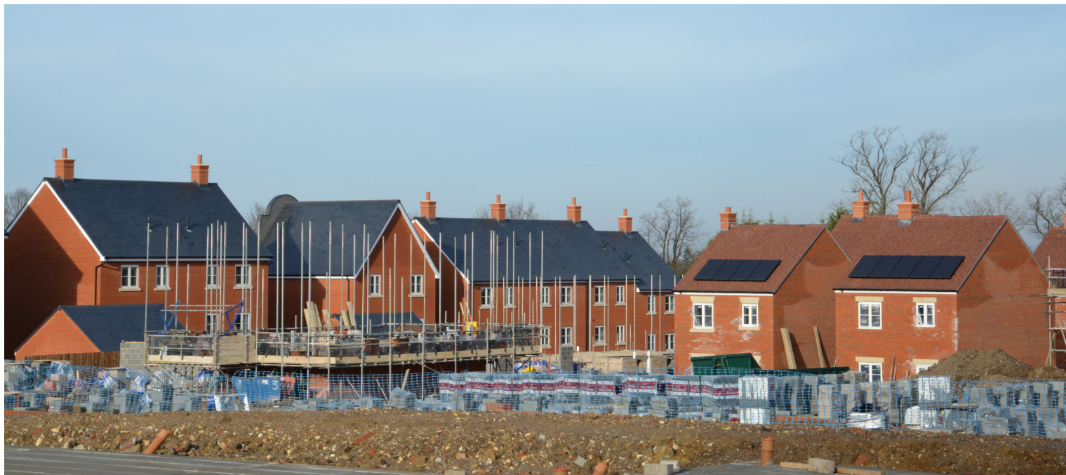
Wellesley's Maida development under construction
